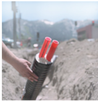
Figure 6, Pex piping
