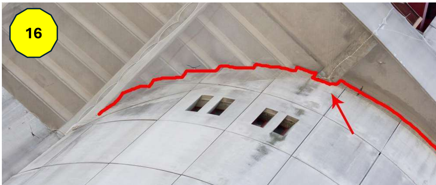
A long slot with accesses for nests and roosts, with a horizontal first trend (from right) and then broken towards the left, sloping in height, to follow the supports of the bleachers. (photo: Milo Manica
